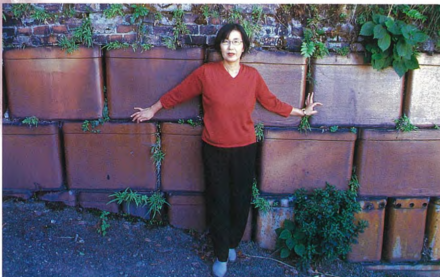
電解槽の土留め Retaining wall of tubs that were once used as insulators for electrical process
